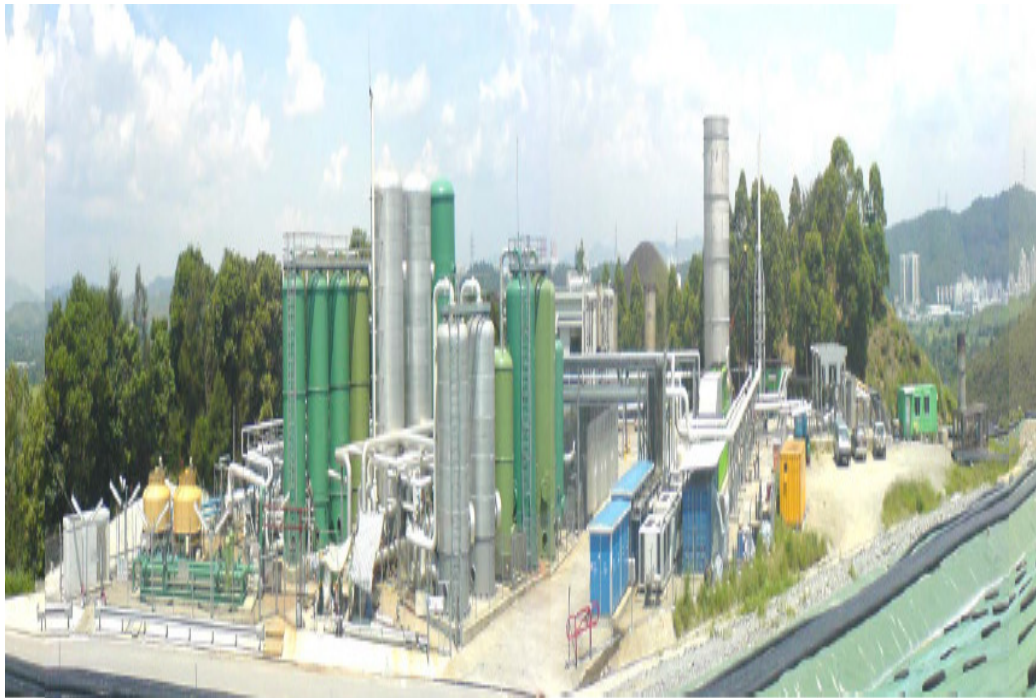
Figure 9: NENT Landfill Gas Treatment Unit
