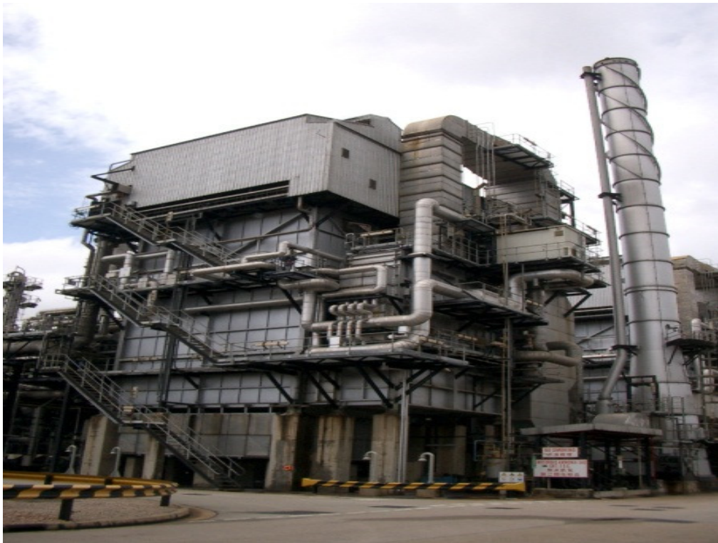
Figure 10: Tai Po Plant Steam Reformer
